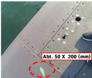
Fig. 5. Delamination of the gel coat during the test.
