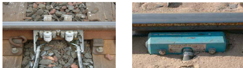
Fig. 3. Sensors installed on the rail
