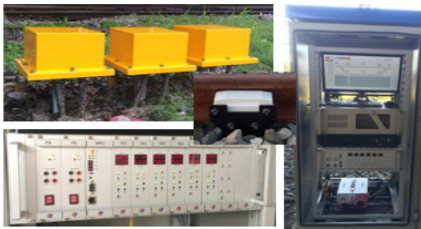
Fig. 8. ACS Pilot Test at O-bong station
