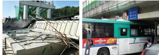
[Fig. 3] PSC beams dropped down from the pier(left) and an accident caused by insufficient clearance(right)
