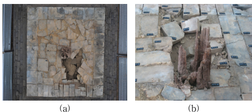
[Fig. 17] Center pole installation(Andong Jotap-ri 5-story brick pagoda Conference Material Reference) (a)Plain (b)Installation status
