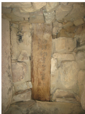
[Fig. 16] Wood pole installation inside 1th floor pagoda body
