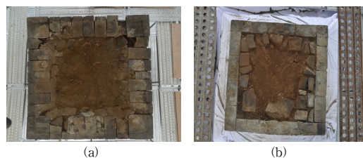
[Fig. 19] Andong Jotap-ri 5-story brick pagoda's interal Jeoksim configuration(Andong Jotap-ri 5-story brick pagoda Conference Material Reference) (a)External wall configuration (b)Buffer zone formation
