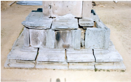
[Fig. 2] Before Breaking up and repairing Gameunsa Temple site(Jang Suk-Ha, Chung Hae-Doo, A study on characteristics of composition method of inner foundation in stone stupa Reference)
