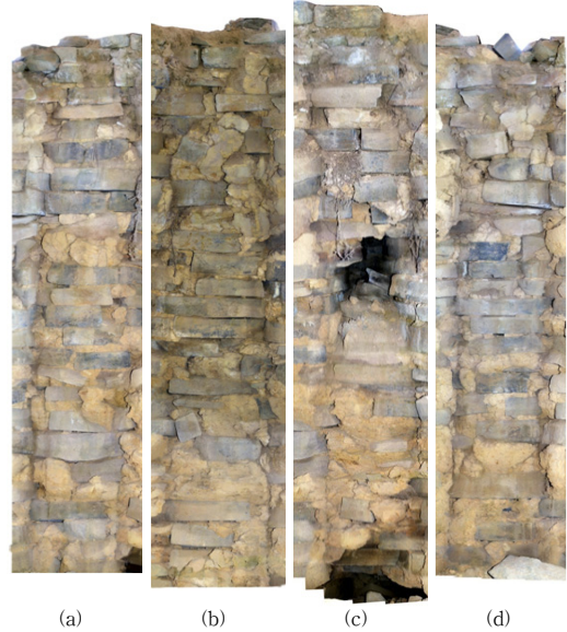
[Fig. 21] Steel pole hole cross section(Andong Jotap-ri 5-story brick pagoda Conference Material Reference) (a)East (b)West (c)South (d)North
