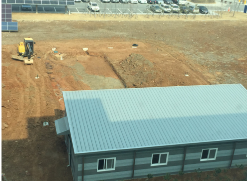
Fig. 11. The scene of cable burying
