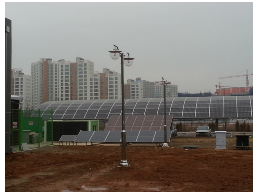
Fig. 14. Installation of streetlight as load
