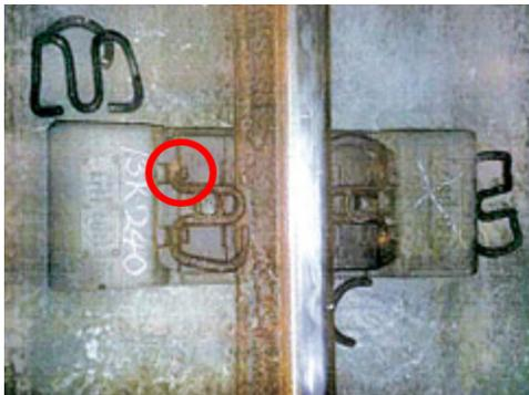
Fig. 1. Damaged Tension Clamp
