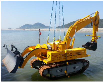
Fig. 1. Underwater equipment for rubble mound leveling
