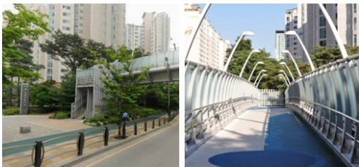
[Fig. 8] Pedestrian Overpass
