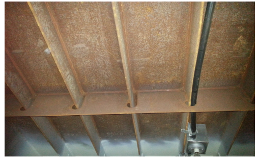
Fig. 5. Box girder (36th span, upper)
