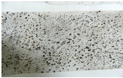
Fig. 9. Box girder (36th span, left)
