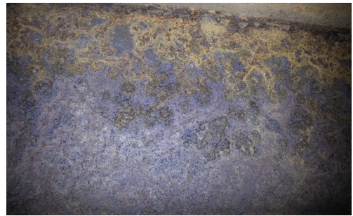
Fig. 6. Box girder (37th span, upper)
