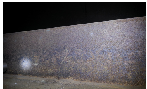
Fig. 8. Box girder (37th span, bottom)
