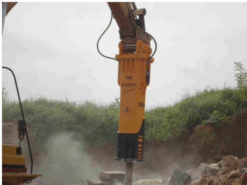
Fig. 6. Picture of hydraulic breaker field test
