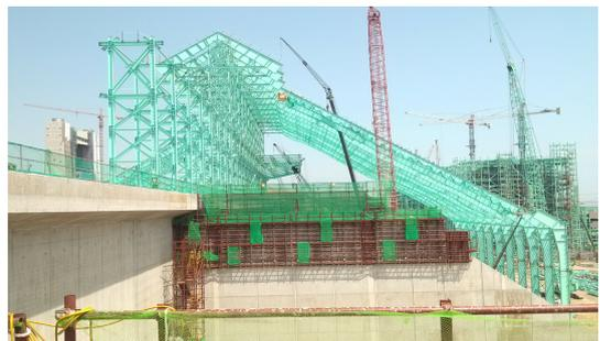
Fig. 5. The site erection of P.E.B. system steel structure
