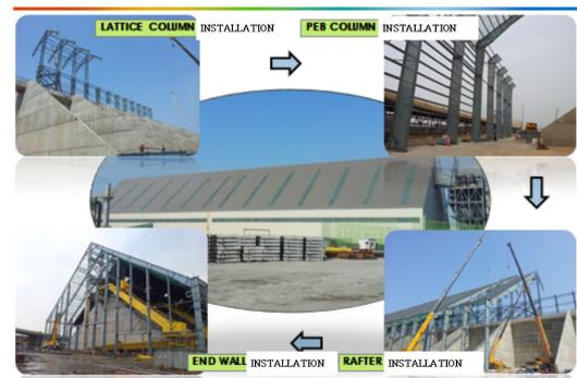
Fig. 4. The steel structure installation procedure of the coal shed
