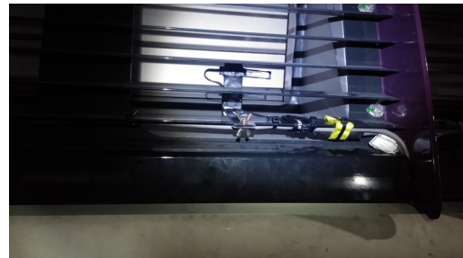
Fig. 3. Installed sensor at upper side grill
