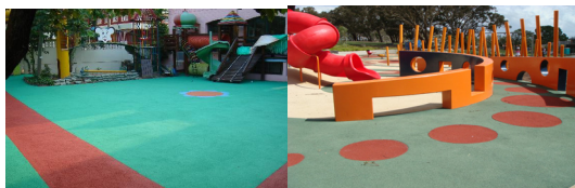
(a) a playground in Korea (b) a park in Australia Fig. 1. Examples of elastic paving
