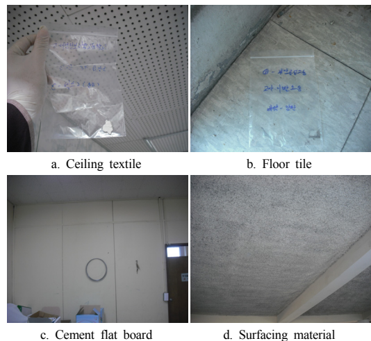
Fig. 1. Survey of ACM at schools
