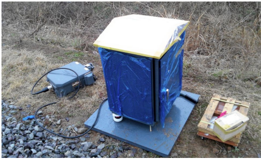
Fig. 3. Installation of switch machine and wayside control unit
