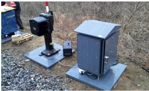
Fig. 4. Installation of crossing gate and wayside control unit
