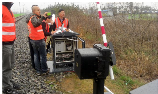
Fig. 6. Fallback control of the crossing gate via LCC simulator
