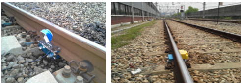
Fig. 3. Installation of the axle counter header
