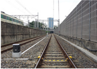
Fig. 14. Installation axle counter sensor
