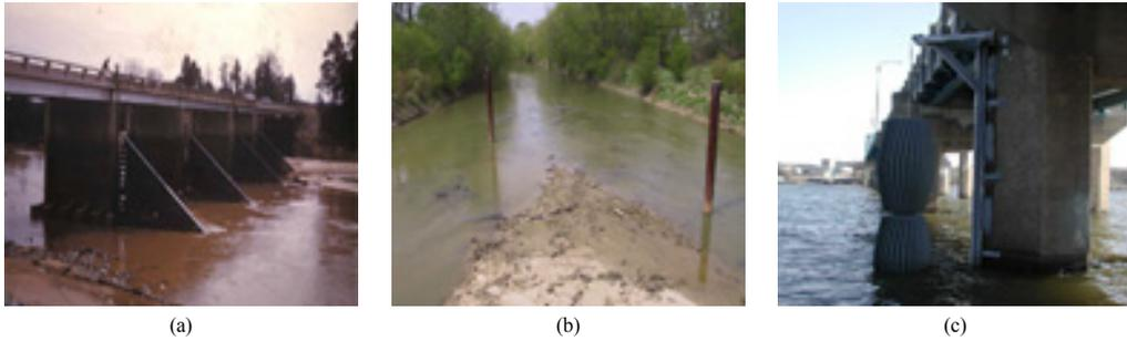
Fig. 1. Debris Deflector(FHWA, 2005)
