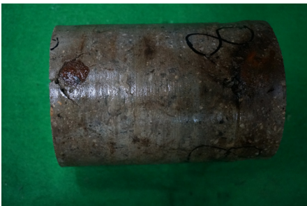
Fig. 1. A cored specimen within a reinforcing bar
