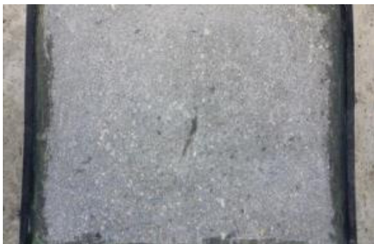
Fig. 15. Surface condition after finishing test
