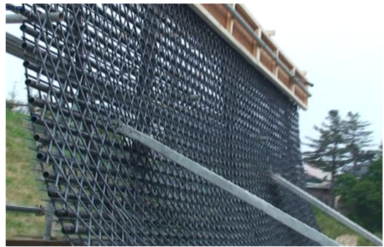
Fig. 2. Foreground of Installed Rebar
