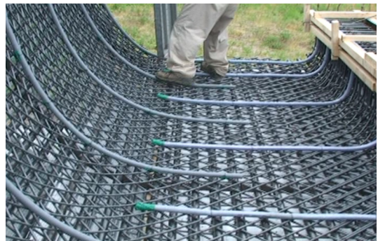
Fig. 3. Foreground of Installed Standard Pipe
