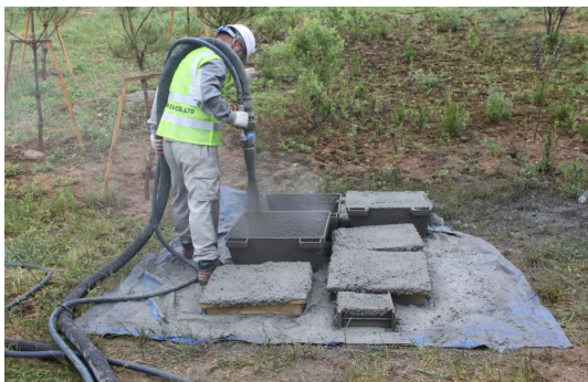
Fig. 9. Molding production for durability test
