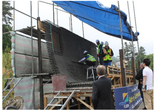
Fig. 10. Screed finishing
