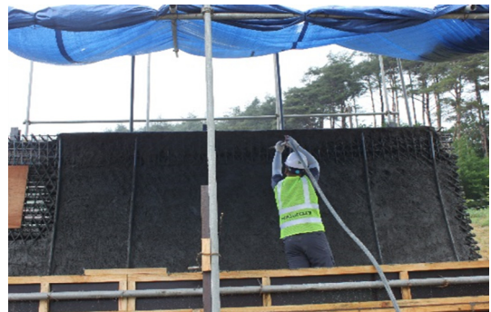
Fig. 6. Rebound elimination using air
