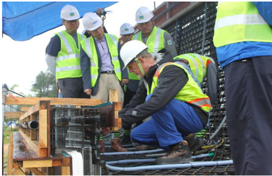
Fig. 4. Reinforced state checking
