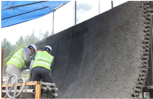
Fig. 8. Placing a secondary surface shotcrete
