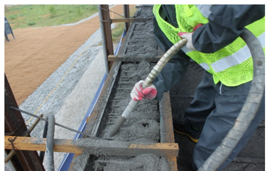
Fig. 7. Vibrofloatation using vibrator
