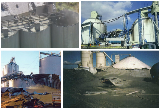
Fig. 2. Examples of silo collapse
