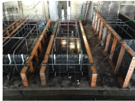
(a) Rebar assembly / Sensor installation
