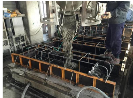
(b) 1 st casting concrete
