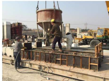
(c) 2 nd casting concrete
