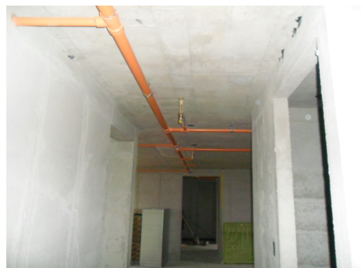
Fig. 5. Construction case of CPVC pipe
