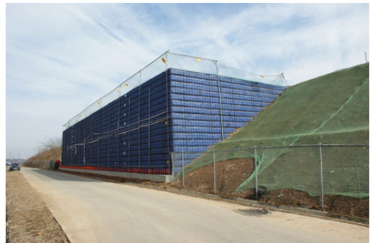
Fig. 6. A view of embankment construction
