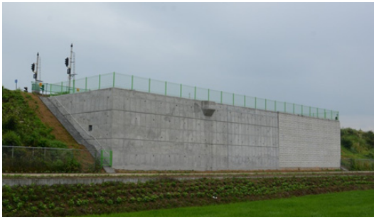
Fig. 7. A view of reinforced concrete wall installation
