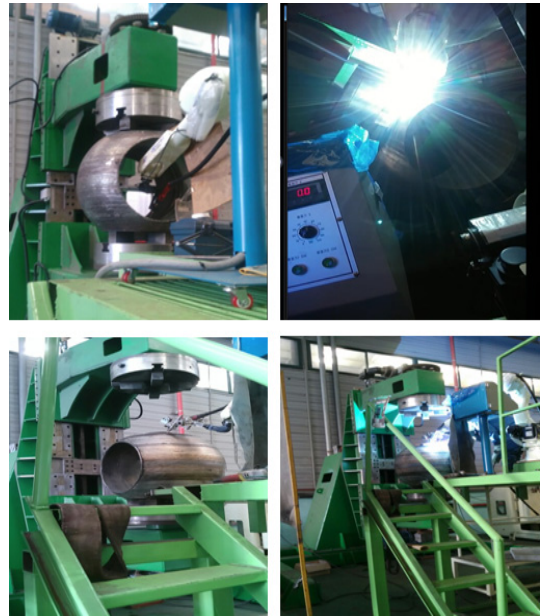
Fig. 14. Operation view of overlay welding by robot
