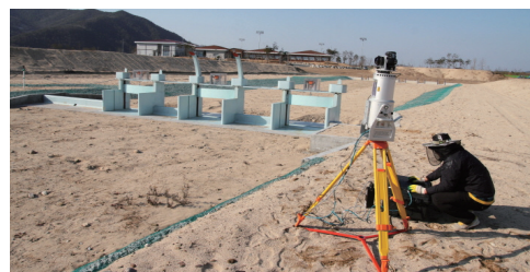
Fig. 4. Scour measurement using 3D scanner
