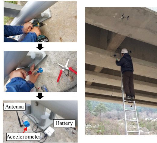
Fig. 5. Installation process of accelerometers
