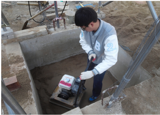
(a) Mockup Chamber and Soil Compaction
