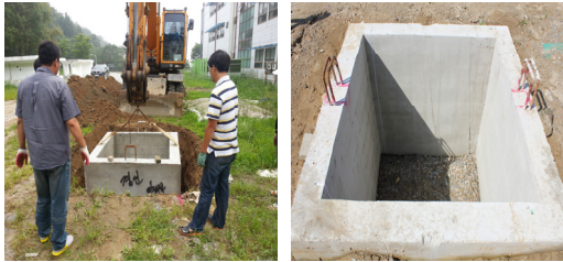
Fig. 2. Mockup chamber installation
