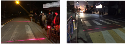
Fig. 6. Recognition light at pedestrian crossing installation view
