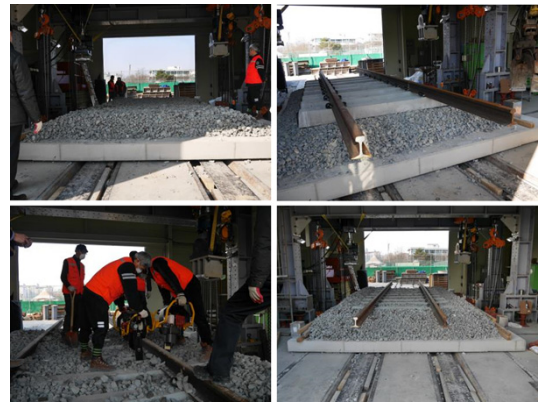
Fig. 7. Fabrication of track
