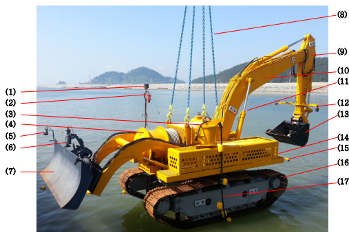
Fig. 11. Composition of underwater equipment for rubble mound leveling(UX-100)
