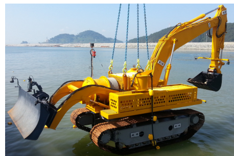
Fig. 5. The underwater equipment for rubble mound leveling(UX-100) [5]
