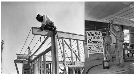
Fig. 1. Cocoon house Construction Photo, 1950
