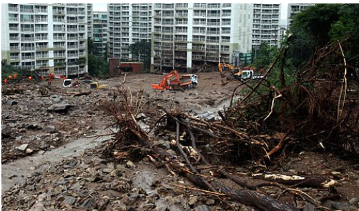
Fig. 2. Umyeon mountain landslide
