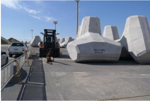
Fig. 3. Dolos2 of 100 tons for repair in Seogwipo port
