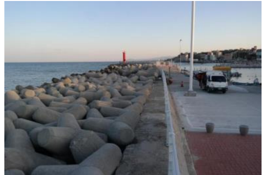
Fig. 1. Armor unit (Tetrapod) in a breakwater
