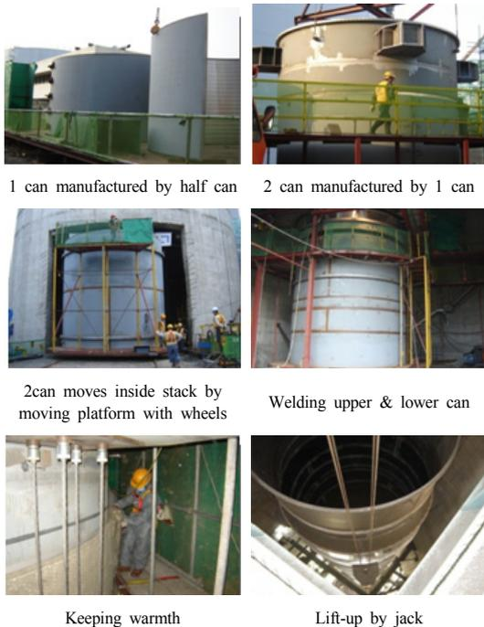
Fig. 11. Installation sequence of steel inner flue
