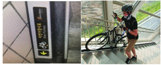
Fig. 9. Example of installation of bike ramp
