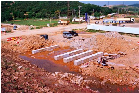
(c) Completion of embankment pile cap
