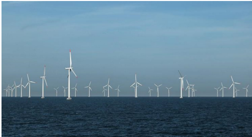
Fig. 1. Nysted Offshore Wind Farm
