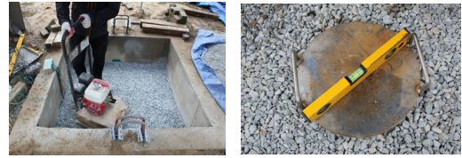
Fig. 7. Ground compaction
