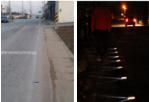
Fig. 7. Rural road safety facility 2
