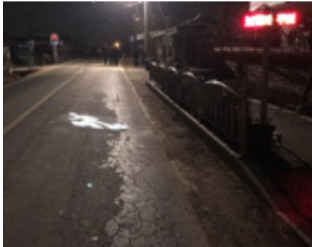
Fig. 9. Improved rural road safety facility 1
