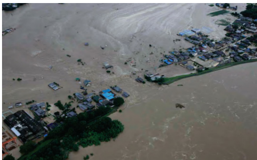
Fig. 1. Levee breach on Kinu river in Japan
