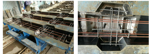
Fig. 4. Arrangement for strands and reinforcing bars at rail-seat section in mold
