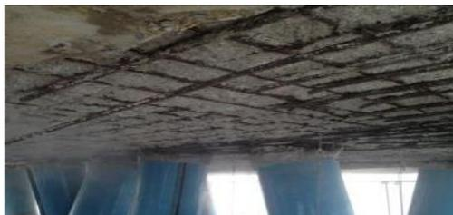
Fig. 2. The Illustration of Harbor Structures Concrete Deterioration [1]
