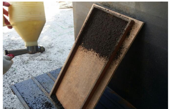
Fig. 1. Installation of green soil
