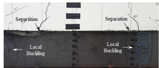
(a) Buckling of Steel plate and separation of concrete slab and deck
