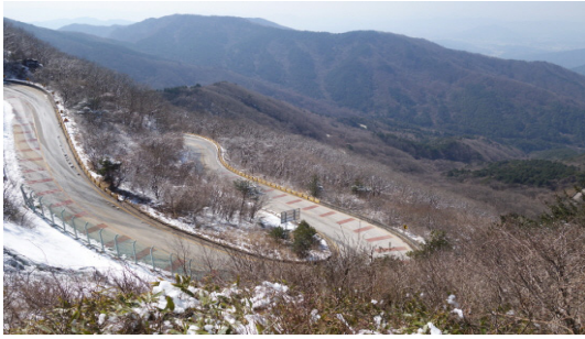
Fig. 3. Steep and sharp curves in mountain roads
