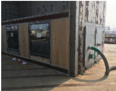
Fig. 3. Air Leakage test
