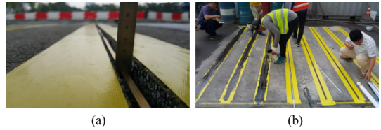
Fig. 8. Traffic sensor installation 2 nd stage (a) Attached the sensor (b) placing the resin
