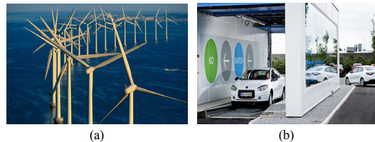
Fig. 7. Copenhagen's Alternative Energy (a) Middelgrundten Wind Farm(middelgrundten.dk) (b) Electric Vehicle(plugincars.com)
