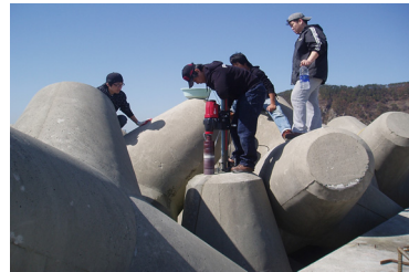
Fig. 5. Extraction of concrete core sample
