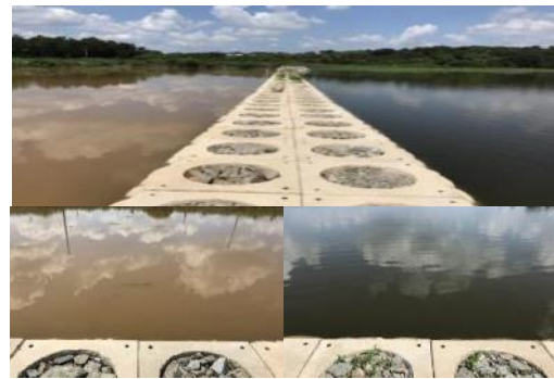
Fig. 2. Secondary dam for water purification
