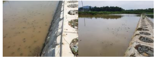
Fig. 2. Secondary dam for water purification
